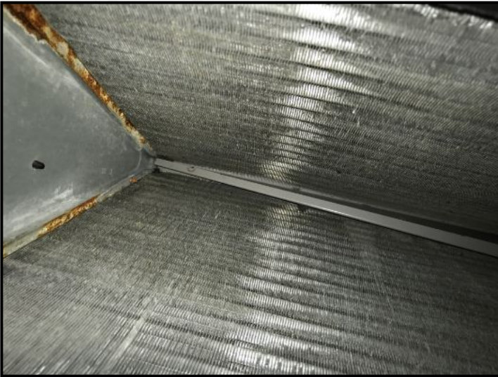
Evaporator coils on the downstairs unit are clean
