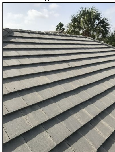
Slipped tile. This is in the area that has the leak above the garage. I doubt this is the main cause of the leak. Most likely there is damage to the flashing underneath.
