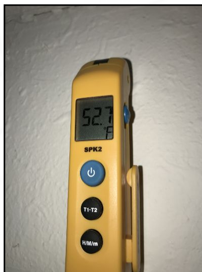
Cooling temperature for the upstairs unit was 52.7 degrees
