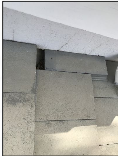
Slipped tile. This is in the area that has the leak above the garage. I doubt this is the main cause of the leak. Most likely there is damage to the flashing underneath.
