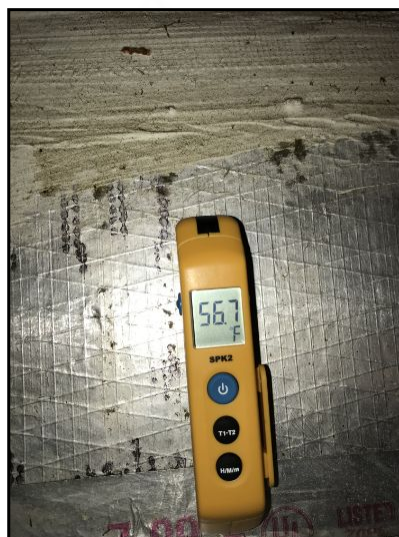
Cooling temperature for the downstairs unit was 56.7 degrees
