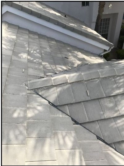
Cap tiles need to be re-mortared
